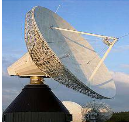
Figure-1: Transmission Antenna
